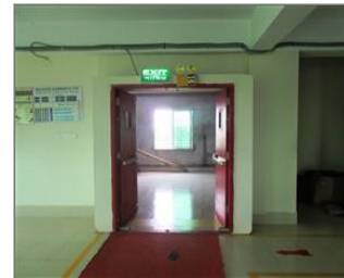
Photo of fire safety equipment Exit sign.JPG
